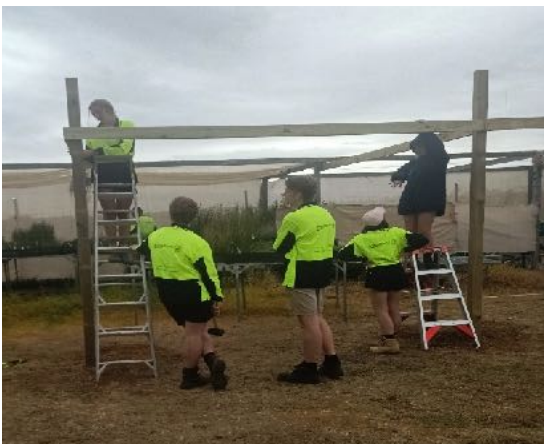
Constructing the Nursery extension
